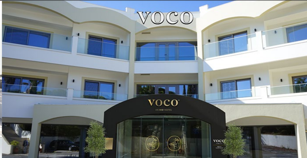
voco Algarve, Portugal – Conversion of the Formosa Park Apartments
